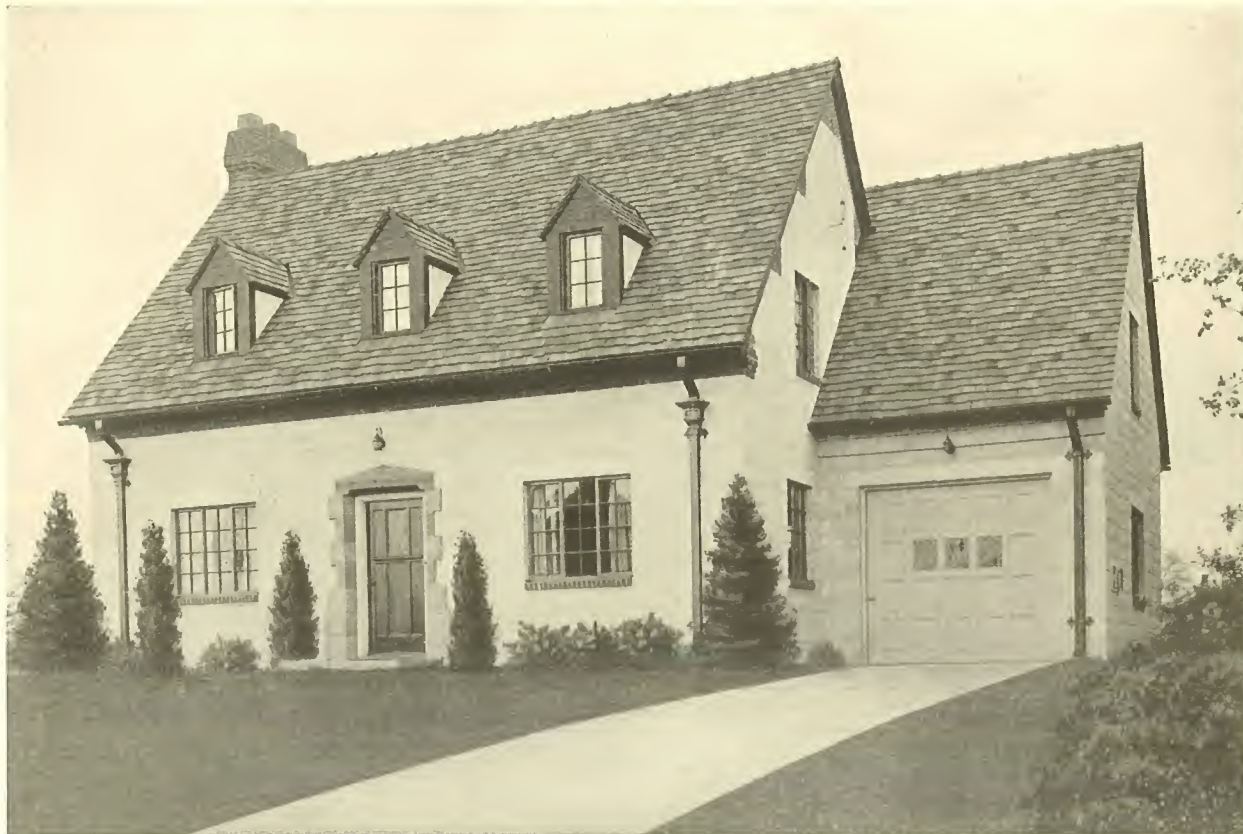
Typical of low-cost, concrete homes is this new Des Moines house with garage attached. The coursed concrete ashlar walls are painted. All floors and partitions are also concrete. Trinsley, McBroom and Higgins, architects.
